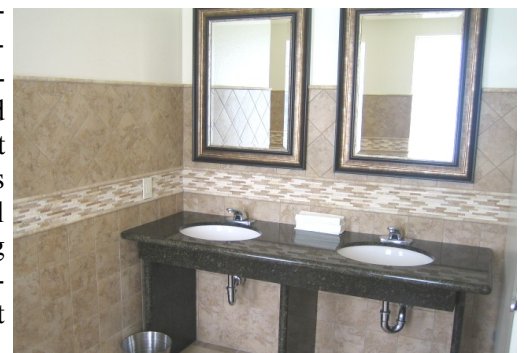
Photo of Remodeled Bathroom
